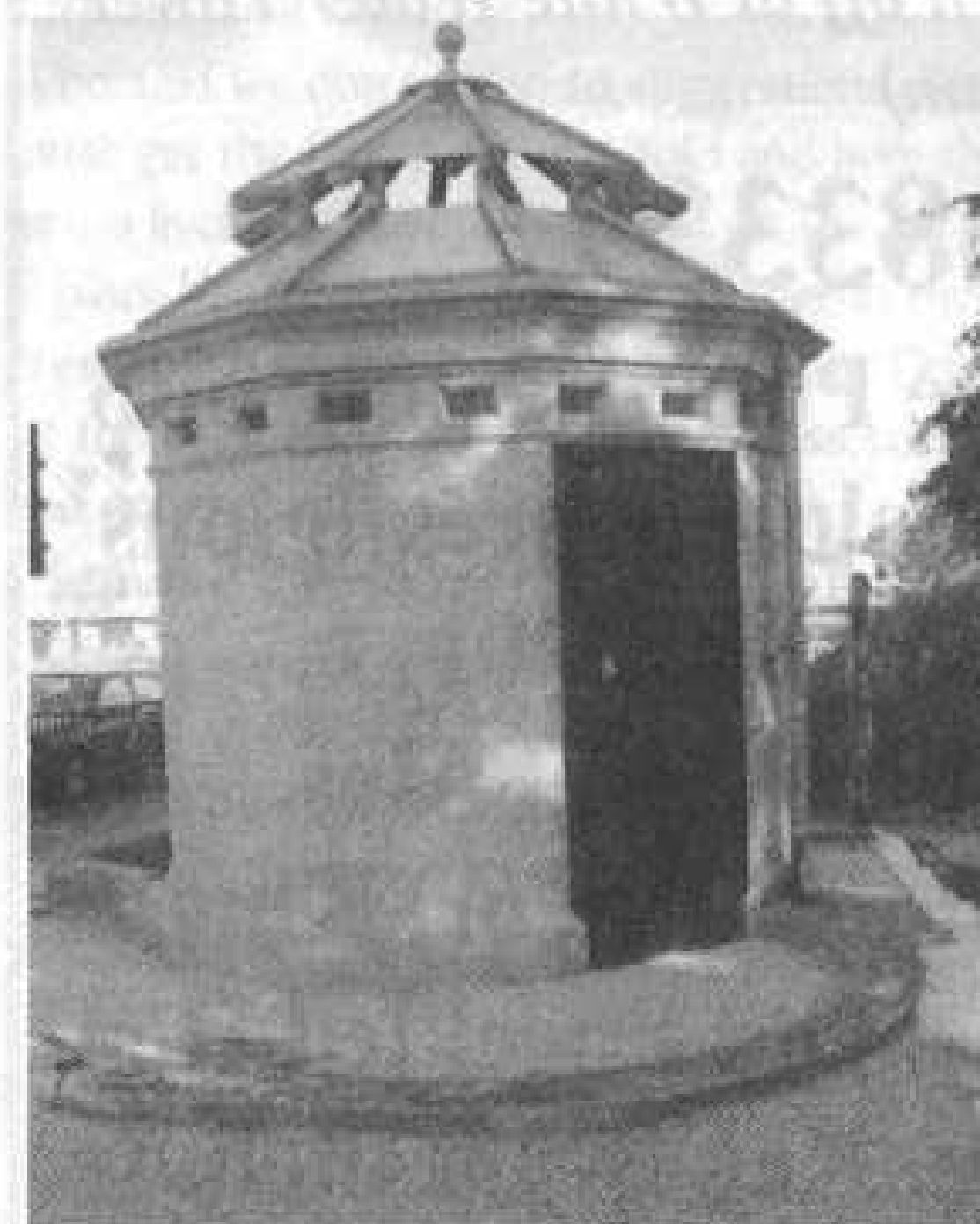
The denuded and rather sad building we are left with now, note original concrete base for the railings
